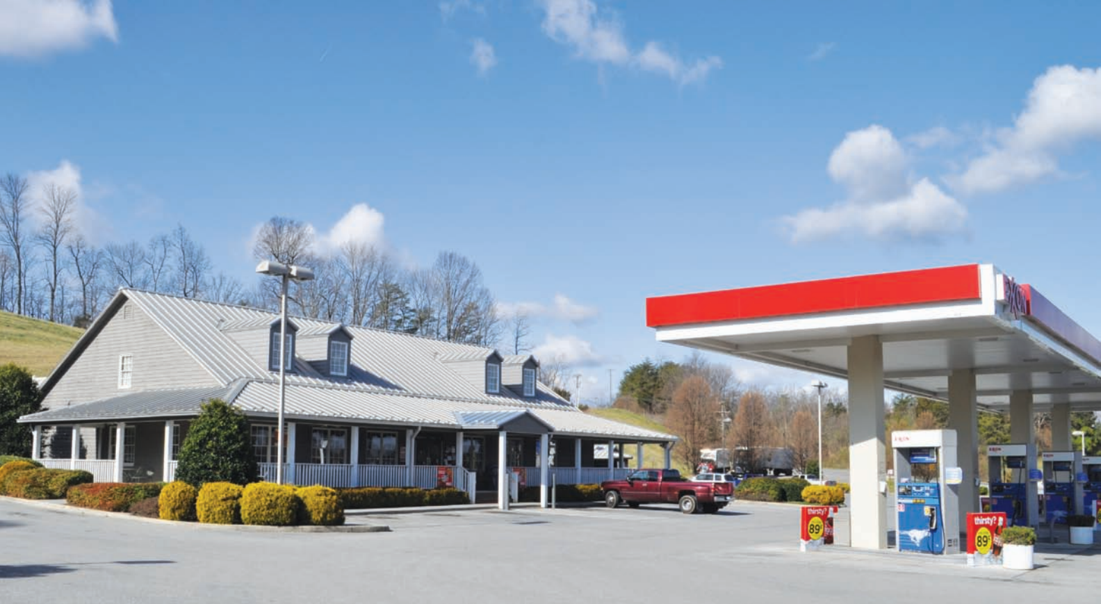
Brugh's Mill Country Store beside I-81
